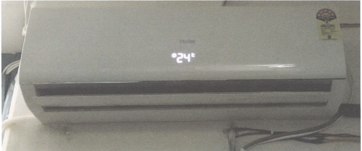
Figure 32 Split type of 5 star,1.5 TR Airconditioning System
