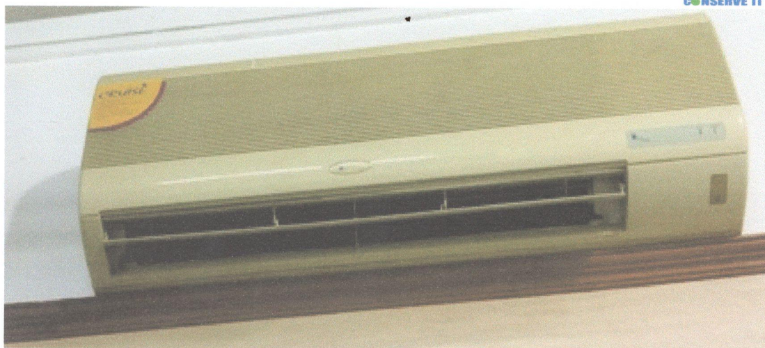
Figure 34 Split type of conventional Old ,1.5 TR Airconditioning System
