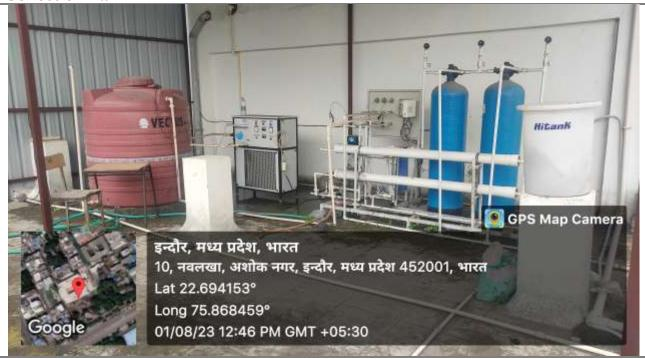
1B. RO Unit Waste Water collected in the **COLLECTION TANK** which is connected to the **flushes of the Toilets** in the Department of Computer Science
