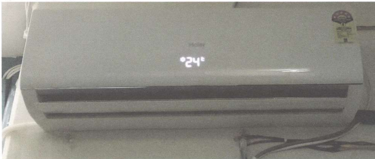
Figure 32 Split type of 5 star,1.5 TR Airconditioning System
